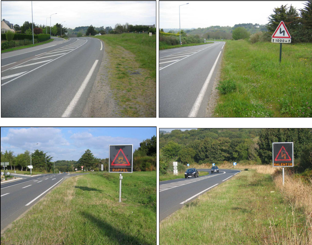
Figure 1: illustration of the information system in curve (above the site without the alert system, bottom the alert system)
