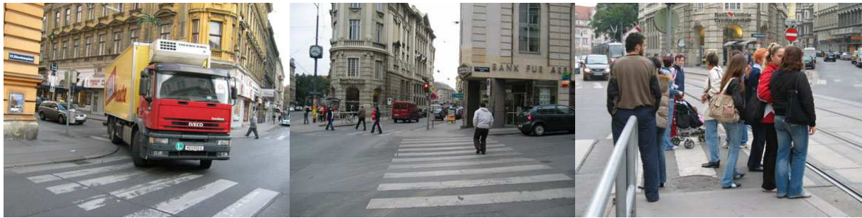
Figure 4: Elterleinplatz before redesign: turning HGV, long crossings, narrow waiting areas
