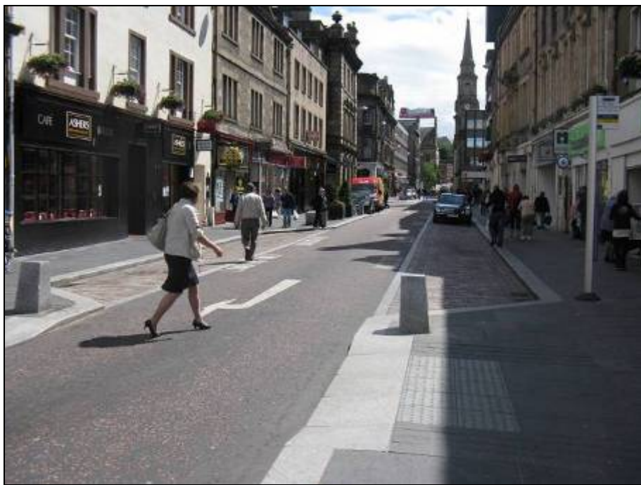
Figure 7: After. Informal crossing as well as formal dropped kerb crossing point, marked with tactile paving (plus kerb build outs providing delineated parking)
