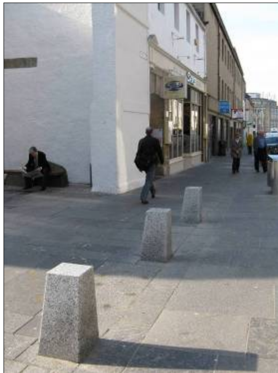
Figure 9: After. Improved materials and public seating
