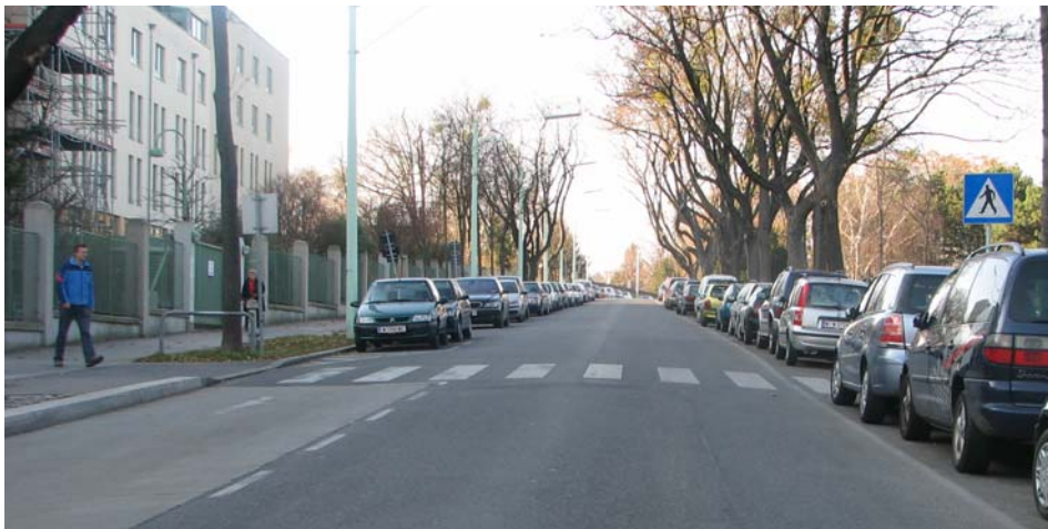
Figure 1 Non-signalised zebra crossing in Austria (minimum standard)
