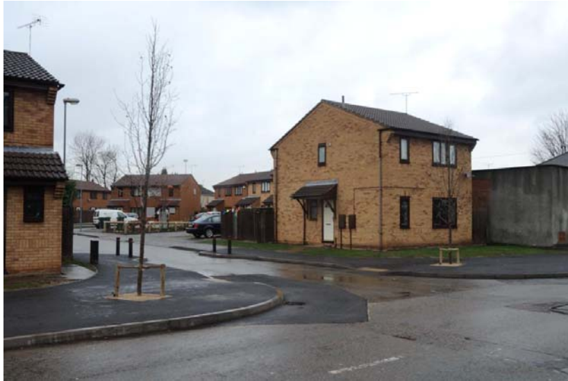
The narrowed junction in Iden Road, Coventry
