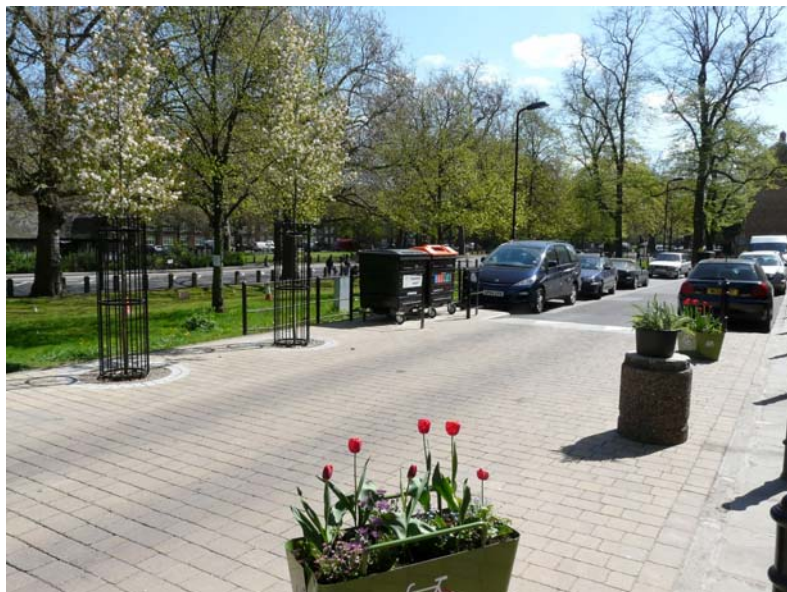
A large speed table becomes a feature of the new design in Clapton Terrace Photo: Adrian Holliday
