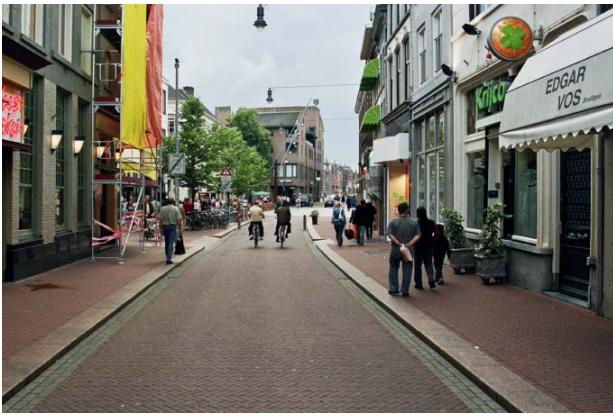
Figure 8/9 Height difference to separate pedestrians from cyclists
