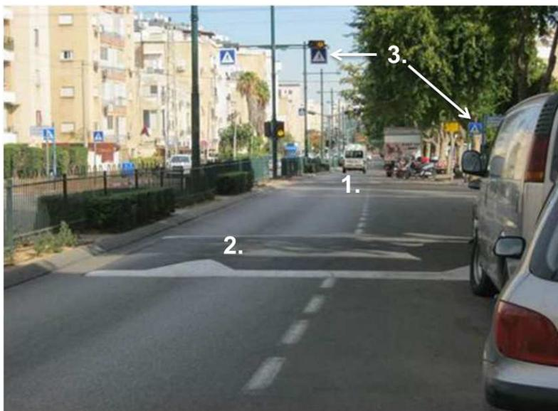
Notes: 1 - a trapezoidal speed hump on the crosswalk area; 2 - a circular speed hump before the crosswalk; 3 – traffic signs and overhead amber flashing lights.
