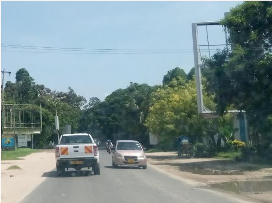
Traffic lanes lacking delineation
