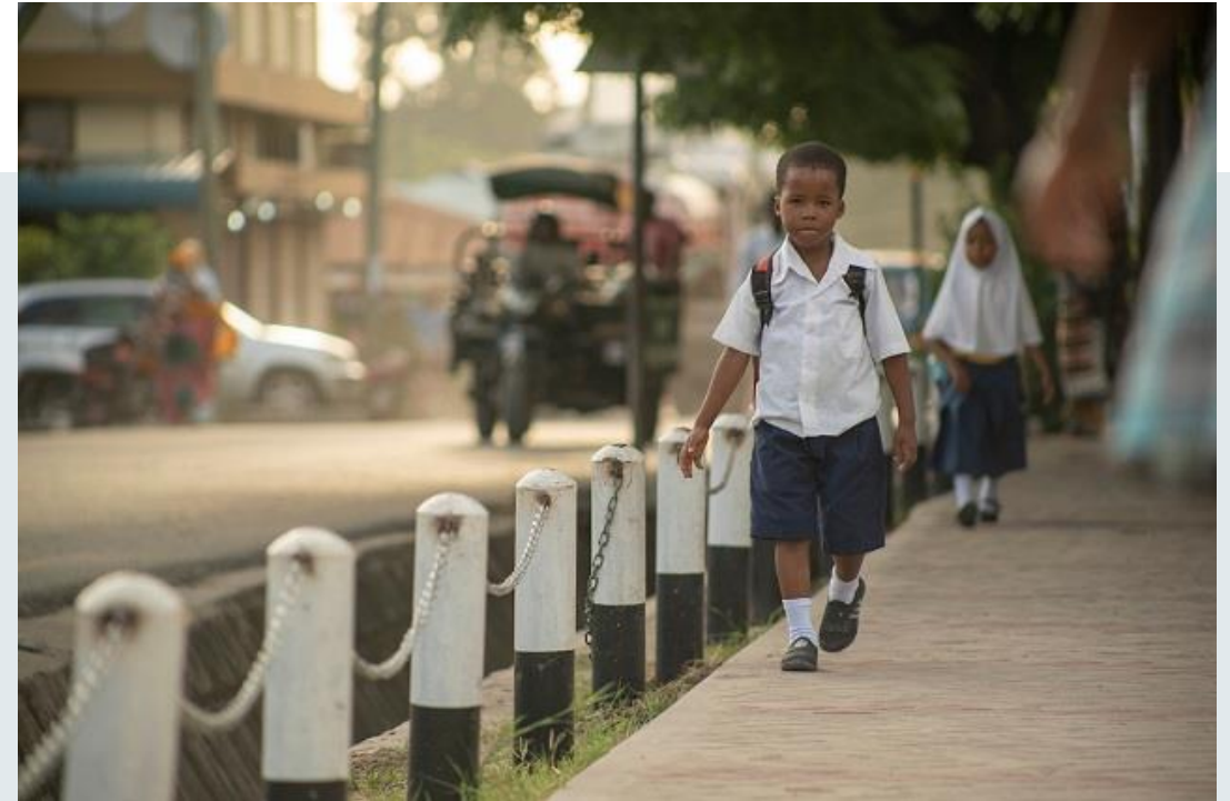
Safe Sidewalk with adequate space and barriers to protect pedestrians
