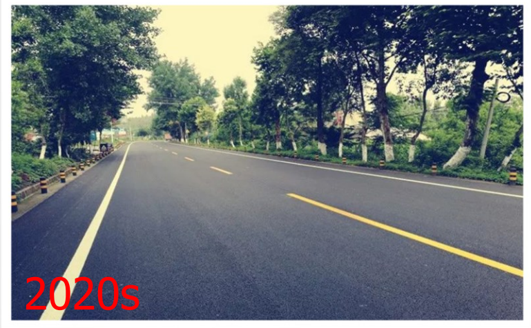
Rural two-lane highway
