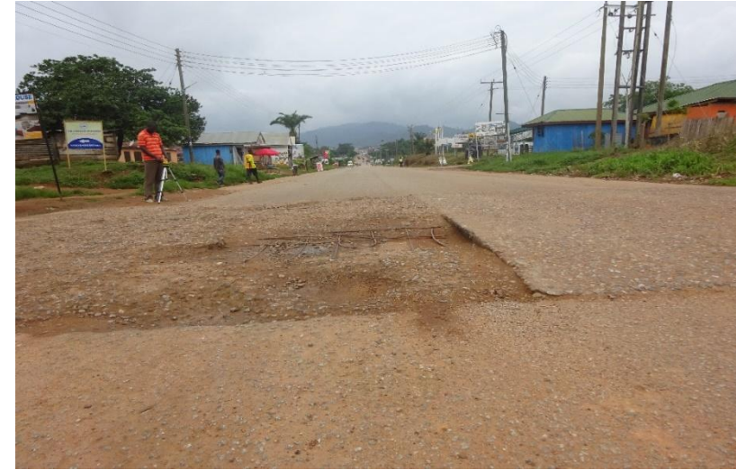
Fig 8: Evidence of speed table deterioration posing road hazard
