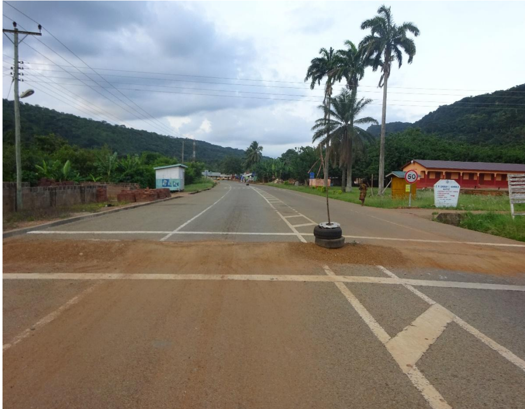
Fig 4: Illegally built speed humps at Matse, Ho
