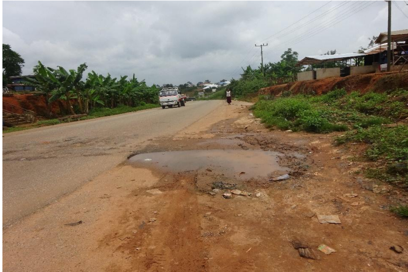
Fig 7: Samples of road deteriorations on pavement- Abuakwa-Bibiani Road
