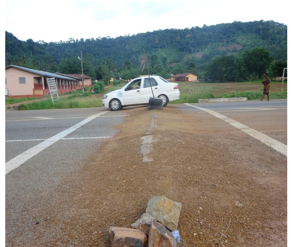
Fig 4: Illegally built speed humps at Matse, Ho
