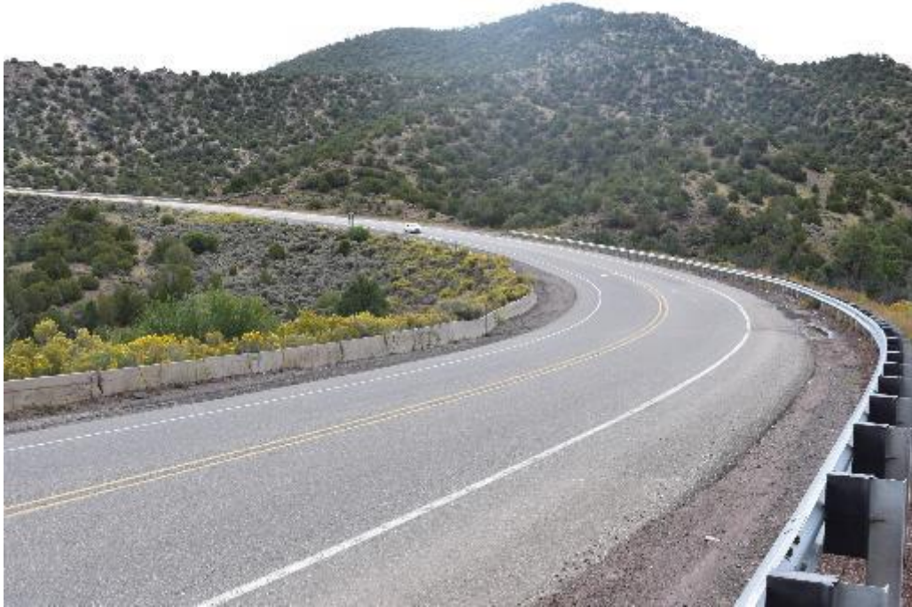
Figure 11 Route 68 Mile markers 32-33 (Google Earth, 2017)
