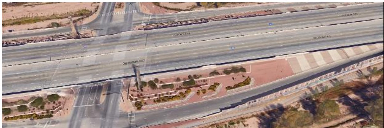
Figure 10 Intersection of Rio Grande and I-40 (Google Earth, 2017)
