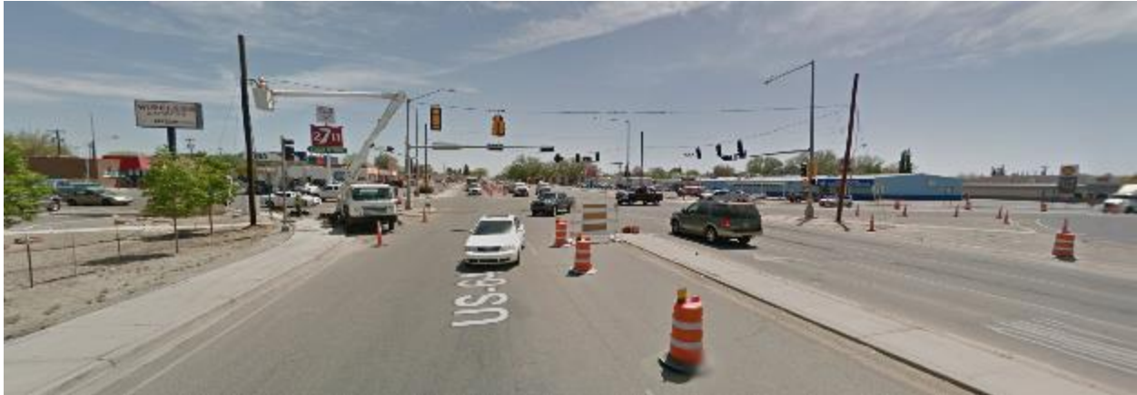
Figure 23 West Broadway Ave Between Church Street and 3rd Street (Google Earth, 2017)
