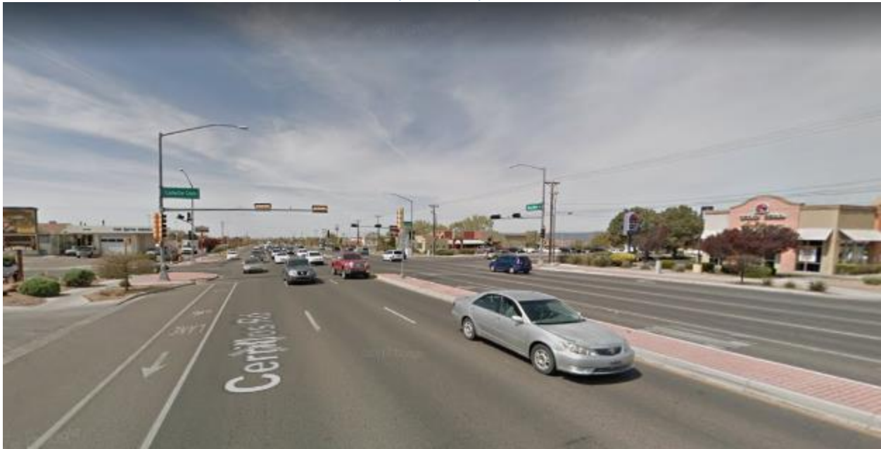
Figure 15 Cerillos Road Mile Marker 50-52 (Google Earth, 2017)
