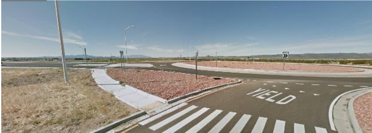
Figure 14 Route 599 Mile Marker 6-7 (Google Earth, 2017)
