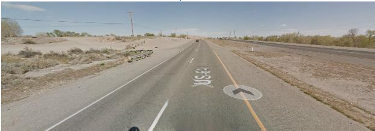
Figure 21 Route 64 Mile Marker 24-30 (Google Earth, 2017)
