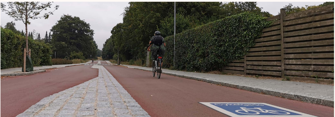
Bicycle street, Højen, Holbæk, with red surfacing and central rain gutters. Photo: Municipality of Holbæk.
