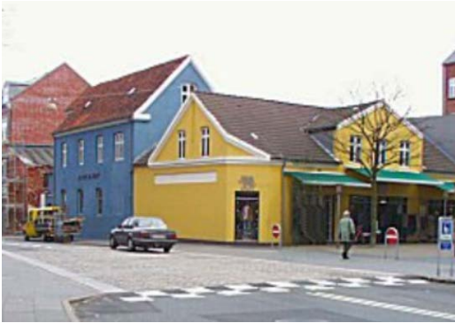
Two-lane raised flat surface at a pedestrian crossing. Photo: Danish Road Directorate.
