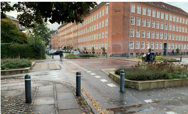
Modal filter with full intersection closure in Guldbergsgade/Sjællandsgade, Copenhagen. Photo: Urban Creators
