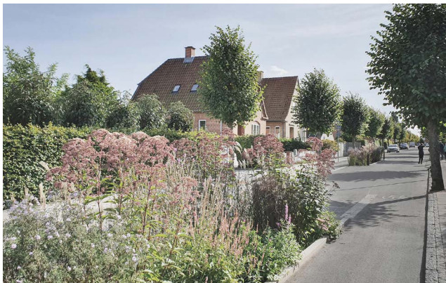
Speed reduction measures in combination with rainwater beds in residential areas in Middelfart. Photo: LYTT Arkitekter.
