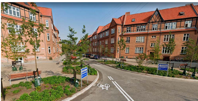
Chr. Kiers Plads (Gerlachsgade/Trepkaskgade), Aarhus. Top: Original design of the intersection. Bottom: The intersection after narrowing and installation of "elephant ears". Photo: Municipality of Aarhus.
