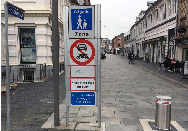
Modal filter with rising bollards at Raupachsgade in Odder. Photo: Municipality of Odder
