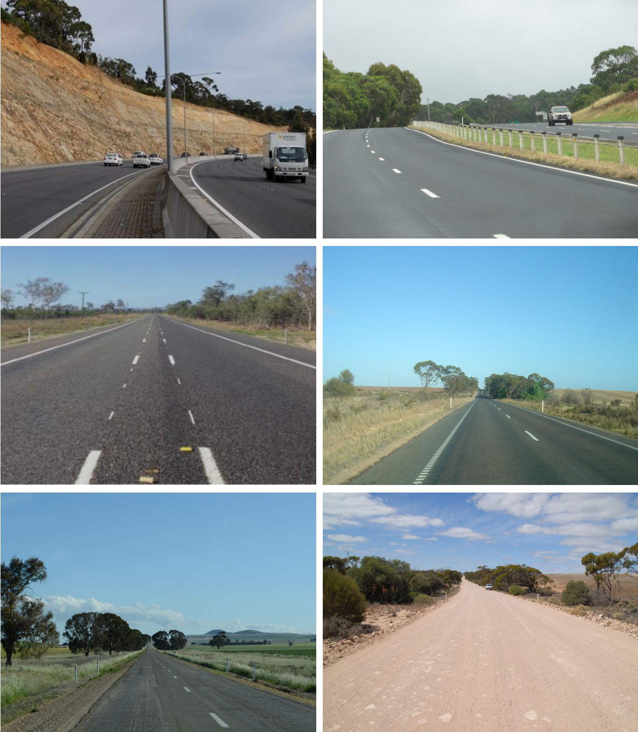
Figure 3.2: Six different road environments all with a 100 km/h speed limit
