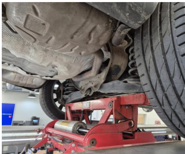
Figure 7: Inspection for corrosion and body structure
