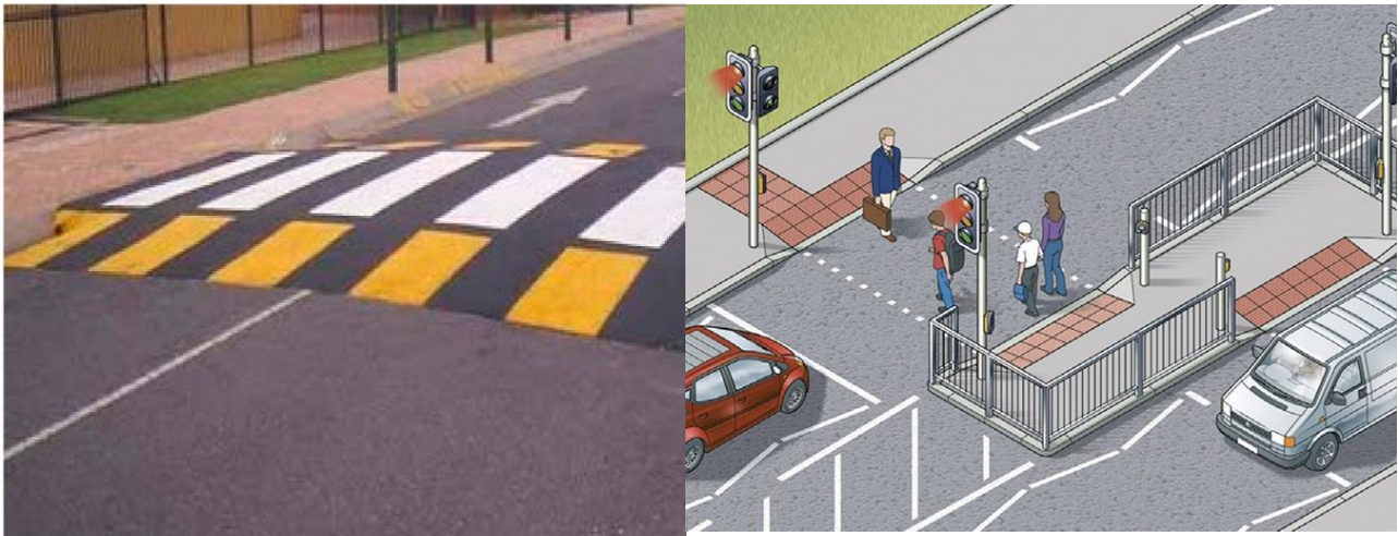
Figure 16. Raised zebra crossing that reduces the speed of vehicles. A staggered pedestrian which allows pedestrians to cross in stages.
