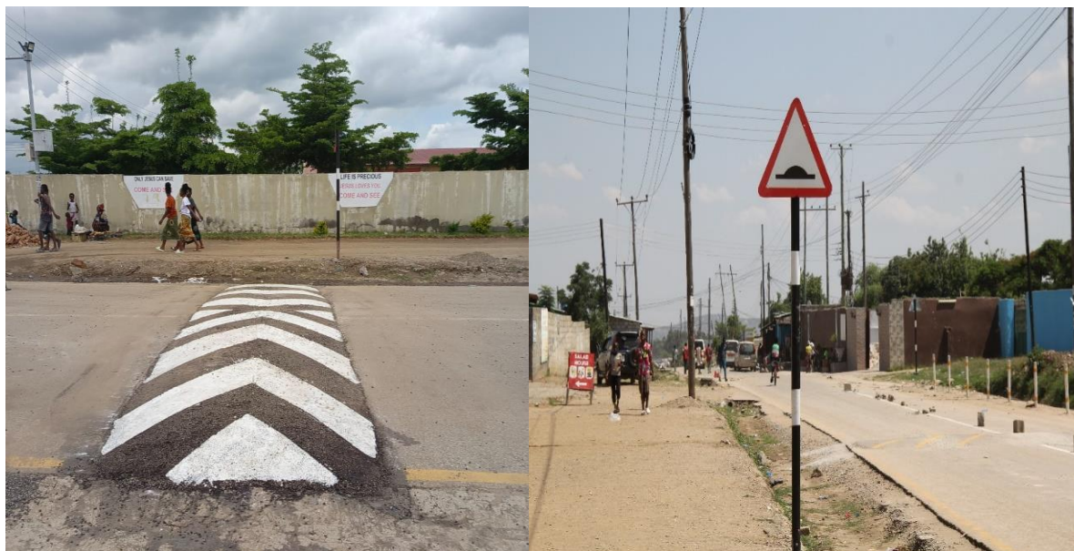
Figure 5. A new speed hump outside Kizito Primary School and a sign to warn vehicle drivers. Photo: Somela Sinkala.
