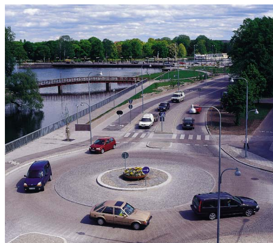
Figure iv: The second major intersection after reconstruction. (Please note that the pictures are taken in opposite directions.)
