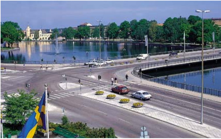
Figure i: The major intersection at Hamngatan before reconstruction.
