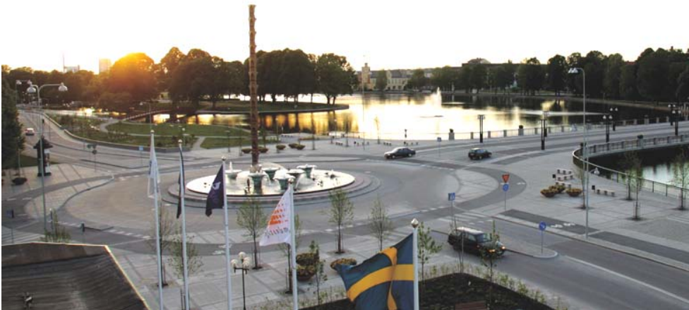
Figure ii: The major intersection at Hamngatan after reconstruction.
