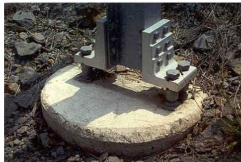
FIGURE17 Breakaway Foundation Stub
