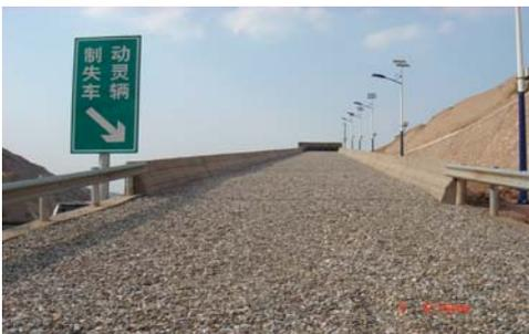
With the investigations and researches by crash frequent points(Table 1), we suggest to set up escaping ramp in K17 400M K63+400M and K65+780M.
