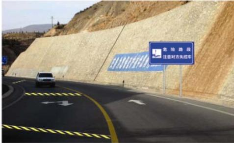
We advise to set up speed control devices on the two side of tunnels' downhill road, the form can be adopt decelerate cingulum or Belgium road surface. The speed control devices can force vehicles to keep lower speed.
