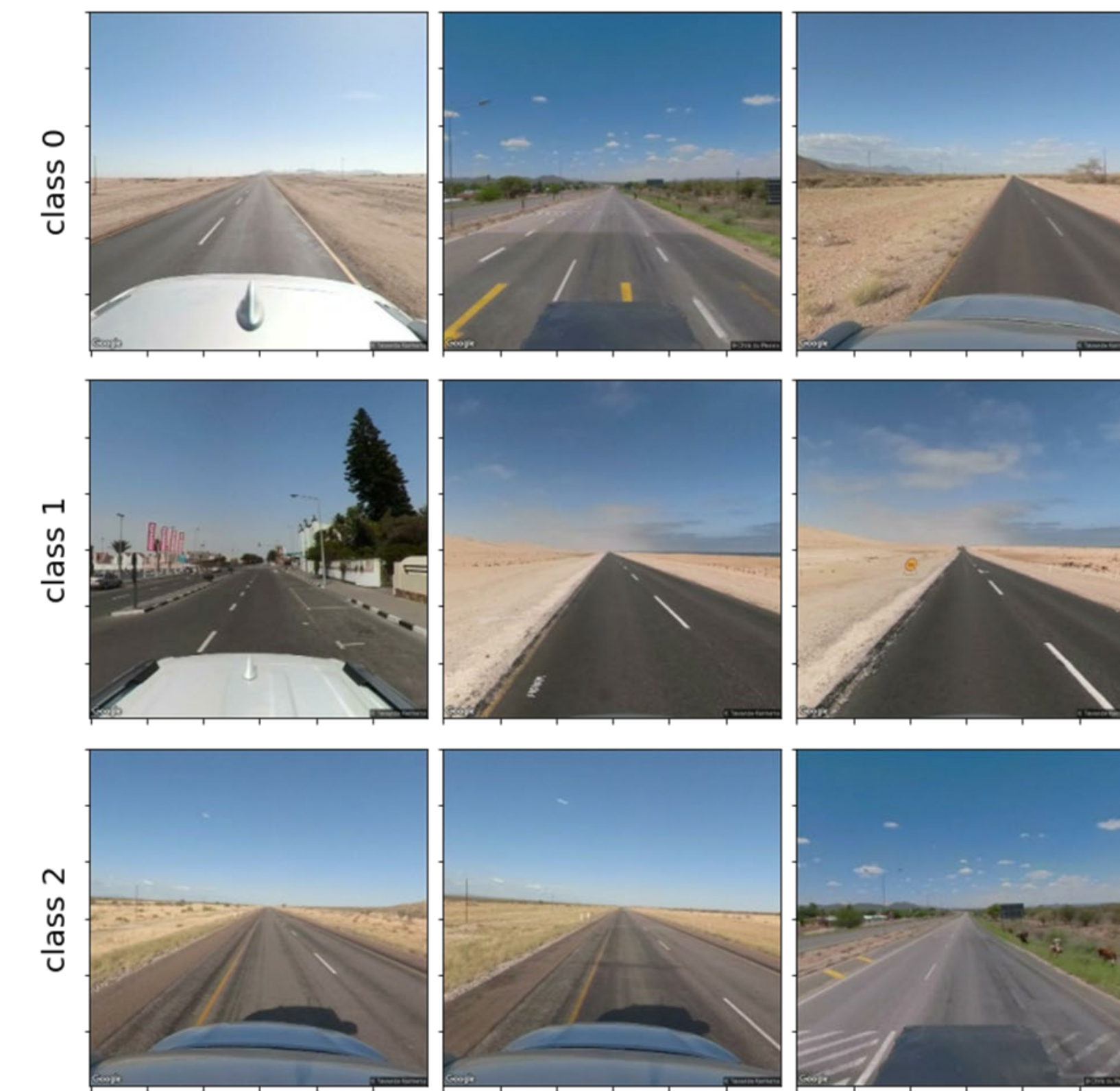
Sample classified road shoulder images. Class 0: no road shoulder; Class 1: < 2 feet; Class 2: > 2 feet.
